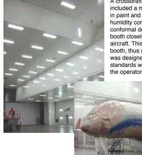
The design for the paint booth was for a 115-foot-wide, 28-foot-high and 115-foot-long room. Exhaust is recirculated in the curing mode (120°F temperature) to reduce energy costs. This booth has five indirect fired air replacement units with direct steam injection for humidity control. The booth is equipped with 3-stage NESHAP filtration. Lighting in the booth is exceptional and rates over 100 fc in most places.
