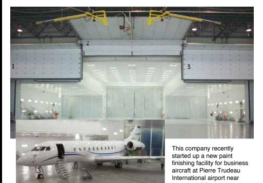
Montreal, QC. A crossdraft paint booth was ordered, and included a multi-mode control system to operate in paint and cure modes with temperature and humidity control. The booth was designed with conformal design, meaning the shape of the booth closely conforms to the shape of the aircraft. This method reduces total airflow in the booth, thus reducing energy use. The booth was designed to achieve high quality finish standards while protecting the environment and the operators.
