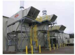
As air is exhausted from process equipment, heat is lost as well. Heat recovery systems are the answer to reclaiming some of the heat that escapes with the exhausted air, in turn providing measurable energy savings. On average, energy recovery systems provide 40-50% energy savings for air make-up systems serving the booth for both heating and cooling.
