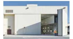
In some instances, such as new building construction, it is better to integrate the paint booth with the building elements. With a Hybrid Aircraft Paint Booth, the structure of the hanger holds up the booth ceiling and the building sidewalls can be integrated into the booth design to economize on material. GFS will work with the building architect(s) to integrate our paint booth design goals with the building design goals.
