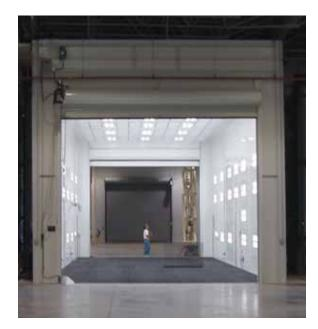
The booth incorporates re-circulation technology and uses filters complying with EPA NESHAP filtration requirements. Filters are located in the basement of the booths via a below-grate stairway. The drive-thru paint spray booths were designed to achieve high quality finish standards while protecting the operators and the environment. VOC and LEL monitors insure safe operator conditions. This complete coating facility is energy efficient and worker safe.
