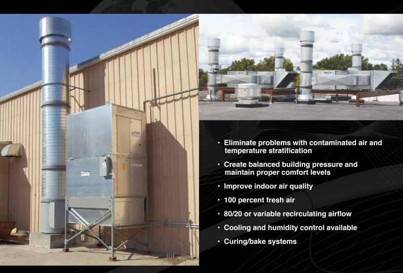
GFS' direct gas fired air make-up units (AMU) provide an economical source of replacement air and are furnished with a heater, filters, motor and blower, controls, mounting hardware and auxiliary equipment. Mounting arrangement options include horizontal or vertical, indoor or outdoor, platform or ceiling suspended.
