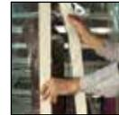
Hook and loop fasteners allow adjacent panels to be easily attached to one another to quickly seal off the work area.
