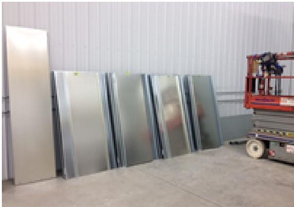
Figure 2. Panels sorted by size in preparation for assembly
