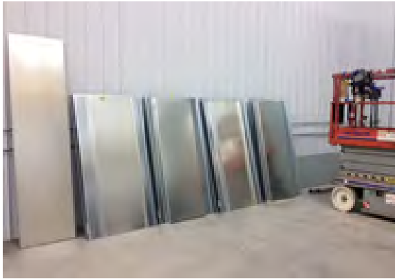
Figure 3. Panels sorted by size in preparation for assembly
