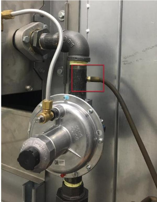
2. Connect the - port of the manometer to sense the low pressure side of the heater box using a T-fitting. The fitting can be located anywhere in the low-pressure line. The manometer is now set up to measure the gas pressure differential across the burner. See Figure 11 on the next page.
