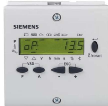
*At left: Flame safety controller built-in display
