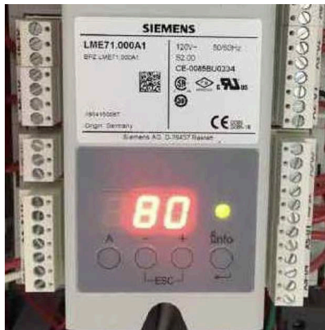
Figure 13. LME7 Siemens flame safety controller
